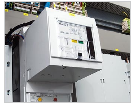
Main switch: An NXM3 circuit-breaker with motor operator also allows remote operation.
