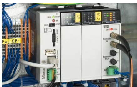
Optimum connection of the XC200 PLC to the welding plant via a local and customised Interbus module
