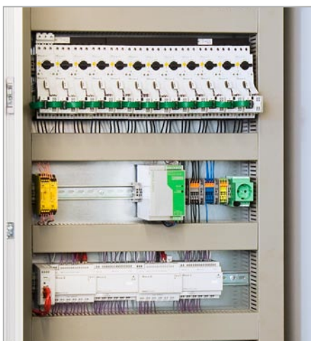
easyConnect SmartWire ensures a "tidy" control cabinet. After all, the control current power supply can be completely replaced with SmartWire.
