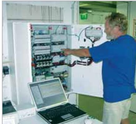
the pools, since, in the event of a failure in individual system sections or modules, the remaining sections continue to operate. In this way, required functions such as the control of water temperature, pool water level, filtering and control of massage jets, as well as the metering of pool chemicals are fully retained.
