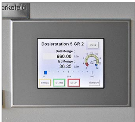
The multi-function display is used to start automated dosing and display the available volume of purified water.
